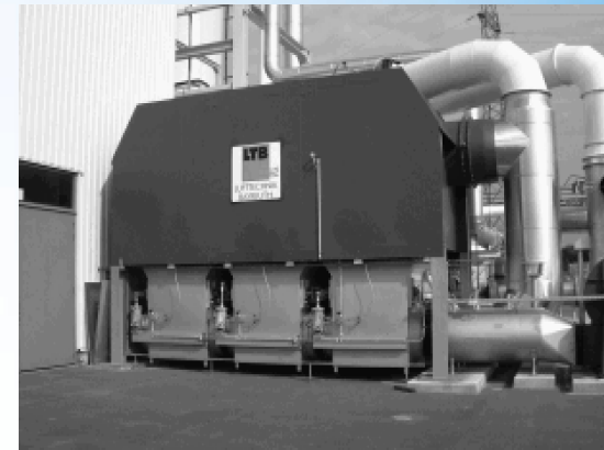
Regenerative purifier with 3 ceramics beds
